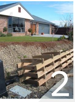
Begin Building Lay the first row of notched components on the concrete foundation, the first two at 200mm centers and the rest at 500mm centers. Lay the first row of horizontal components in the notches, starting with a 1.1 on the front side of the wall and a 2.2 at the back. Continue building the wall alternating horizontal components ie. row 1 starts with 2.2, row 2 starts with 1.1 etc.
