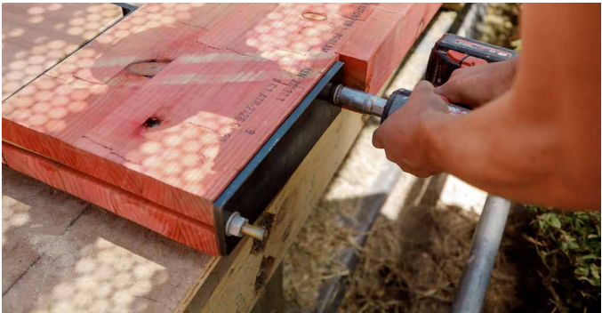
7. Tighten nuts until both curved end plate and conical washers are flattened against the column (to 50Nm Torque).
