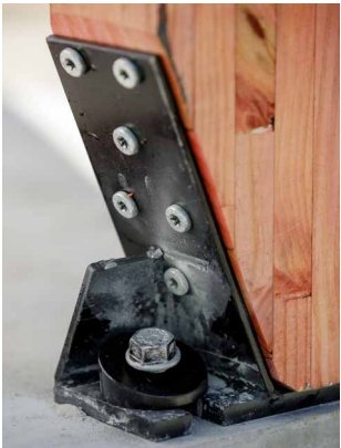
2. For concrete foundations now go to Step 2 to install the foundation connection. For timber sub-floors now add the sq washers and nuts and tighten.
