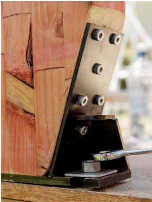
2. For concrete foundations now go to Step 2 to install the foundation connection. For timber sub-floors now add the sq washers and nuts and tighten.
