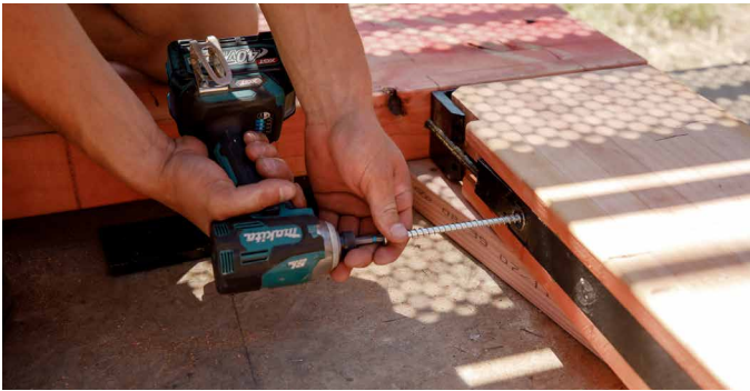
5. Attach dovetail rods with 4x VGS 9x160 screws.
